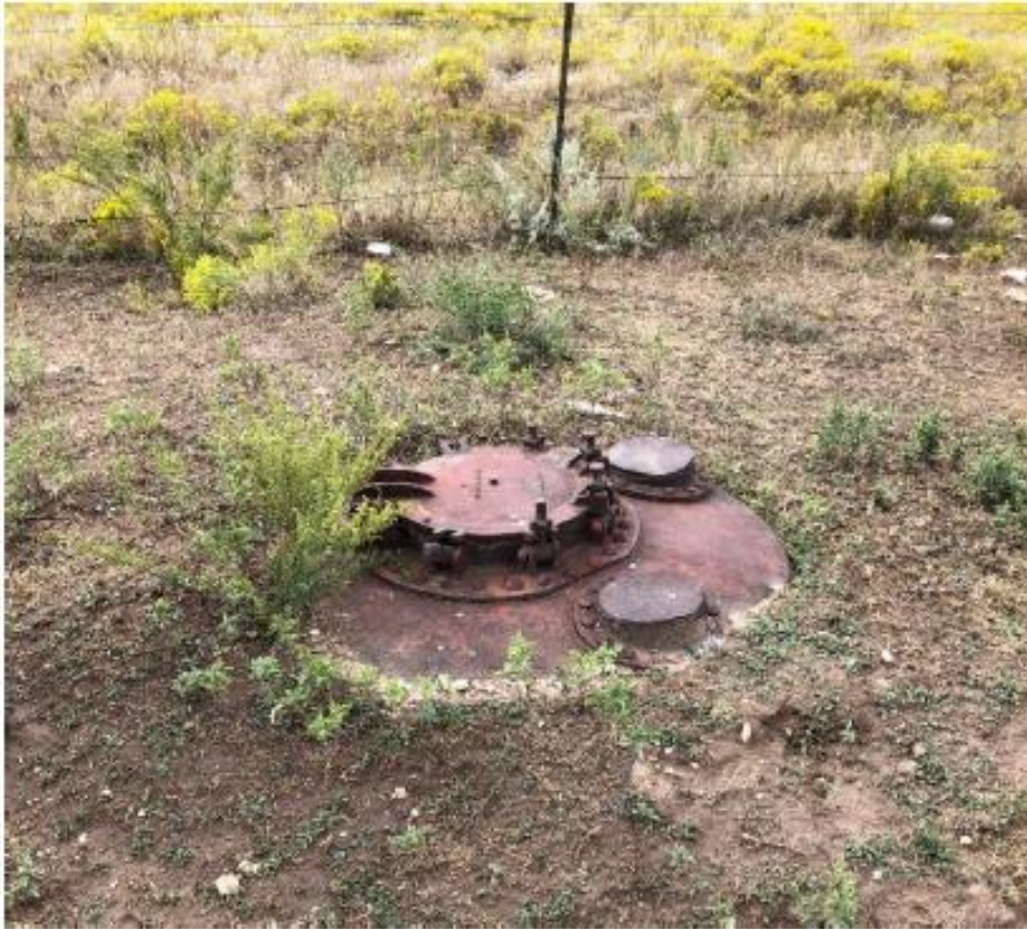
Top of Buried Steel Tank Train Car
